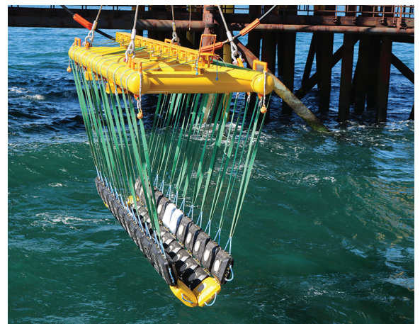
A BOATLOAD OF MATTRESSES WERE NEEDED Luckily, placing them took just 20 minutes each.
