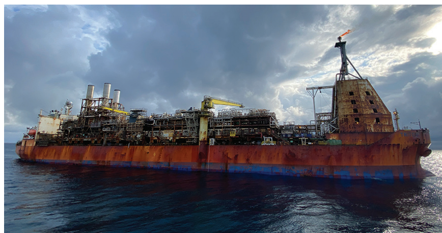
TRITON FPSO The vessel, which sits in 90 metres of water, is 244 metres long and has a storage capacity of 630,000 barrels.
