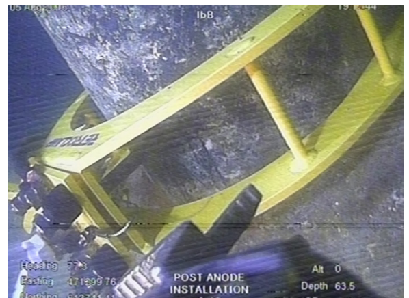
RETROCLAMP INSTALLED ON MEMBER
