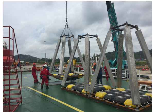
RETROPODS LOADED ONTO VESSEL
