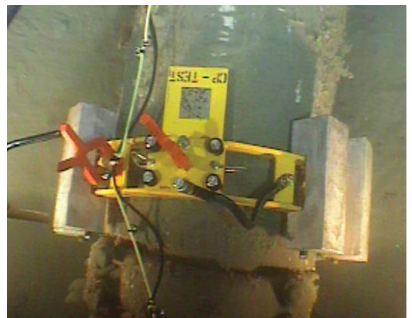
FAST INSTALLATION Most of these clamps were installed in less than an hour each.
