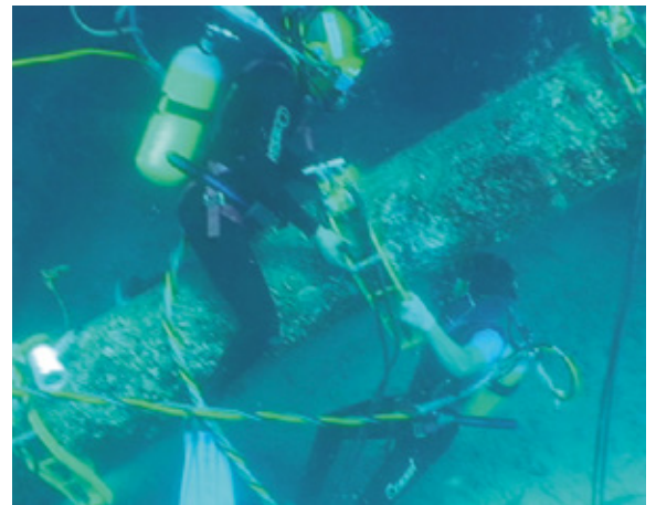
RED SEA RetroClamp on a platform member, connecting RetroPod anode sleds.
